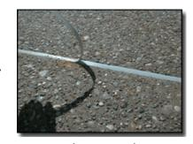
The easiest, most economical way to finish concrete slabs with a water resistant seal. Install KEY-LOC® Joint with our Clean-Strip Cap applied to top edge. Pour and finish concrete slabs. Peel off top of Clean-Strip Cap for the most aesthetically appealing controlled slabs. No need to strip or caulk. #3017 - Clean Strip Cap available in gray and black. Total slab completion in one easy process.
